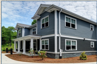
Permanent Supportive Housing
