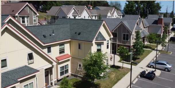
Gordon H. Mansfield Veterans Community, Leeds, MA - 44 Units
