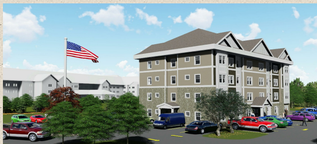
GHM Veterans Community, Tewksbury, MA 21 units – Summer 2024 completion.
